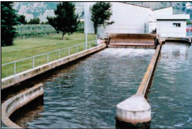
Fig. 4 Ongoing treatment, with FOG control.
